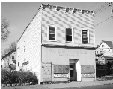
691 E. Third Street was demolished in November 2005 due to a wall collapse. It was the last Italianate wood storefront in the Dayton’s Bluff Historic District. The emergency demolition was allowed through an administrative order signed by the Mayor’s office.
